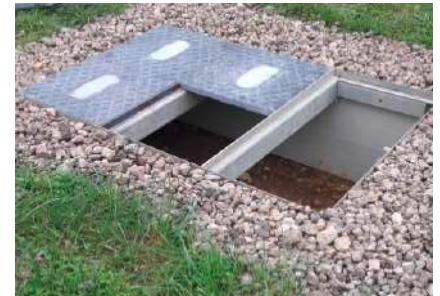
6. The GRP cover plates are installed with a cable junction box lifter.
