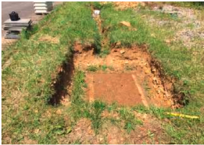
1. Preparation of a stable and even subfloor.
