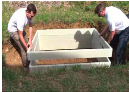
2. Position the first ring and align it accordingly. Then stack the rings on top of each other.
