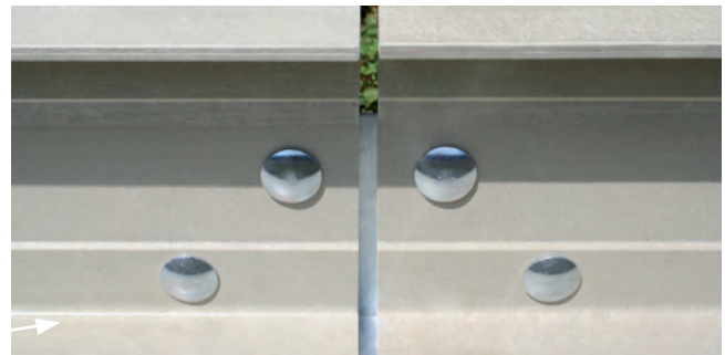
Round headed screws, observed an expansion joint
